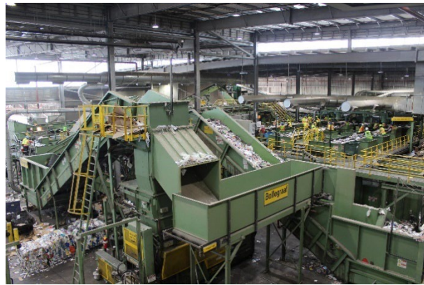
North Gateway Materials Recovery Facility
